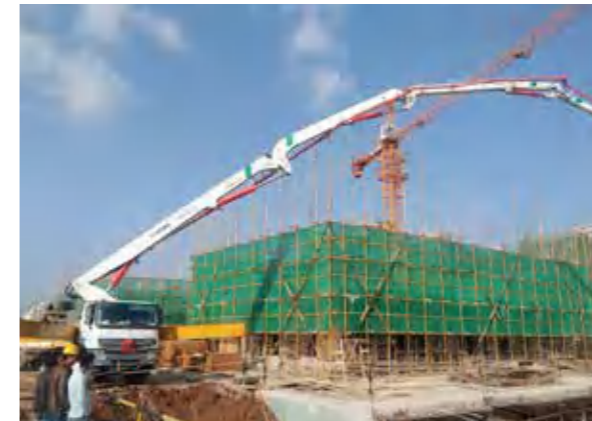
徐工HB52V泵车云南施工 XCMG HB52V boom pump is working in Yunnan
