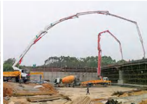
徐工HB62V泵车入驻衡阳 XCMG HB62V boom pump is settling in Hengyang
