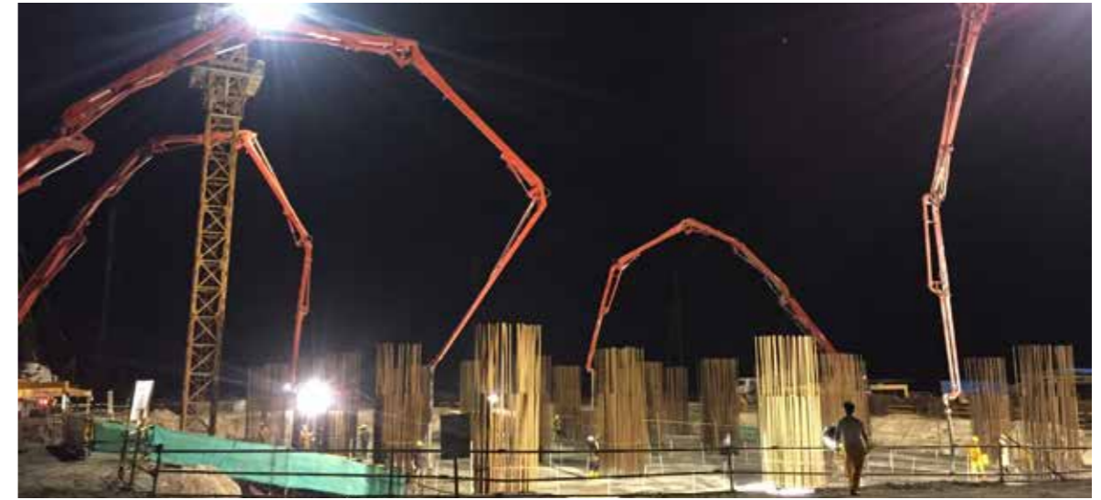
四蛟龙齐助尼日利亚建设 Four boom pump are cooperating like dragons in Nigeria
